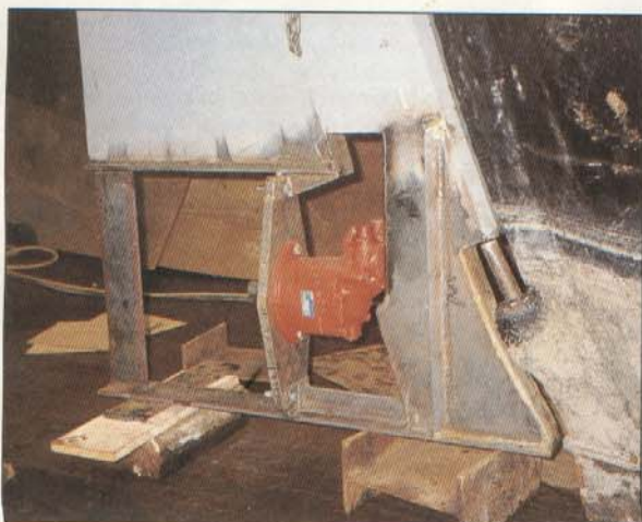
● Detail of the foot of the 'ellum showing the ARS hydraulic motor before the hydraulic pipes were fitted.
